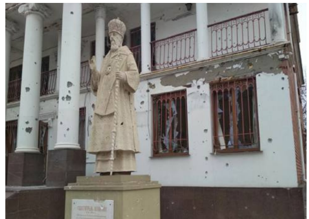
The damaged monument to Saint Metropolitan Ignatius, one of the founders of Mariupol, in the yard of the Greek cultural centre “Meotyda”
